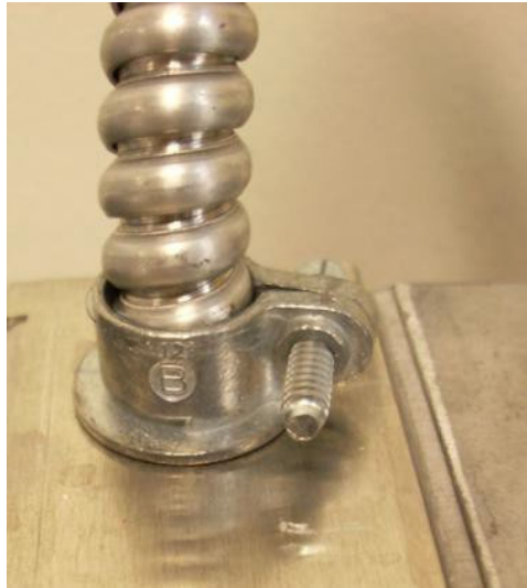
Figure 6: Non-Ferrous Fitting on Junction Box (not user serviceable)
