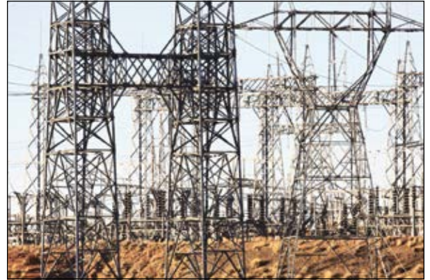
Power sources are especially vulnerable to EMP and IEMI events. The resulting indefinite loss of power and communication will be catastrophic to government and society.
